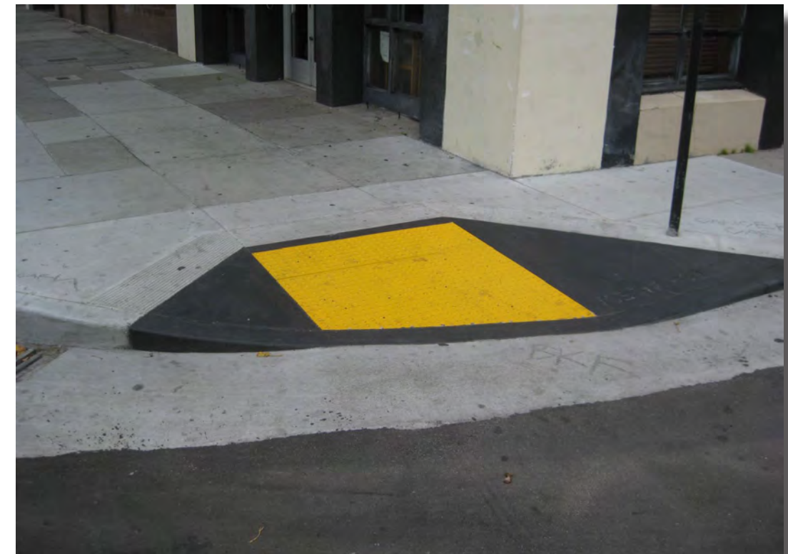
Example of an ADA curb ramp
