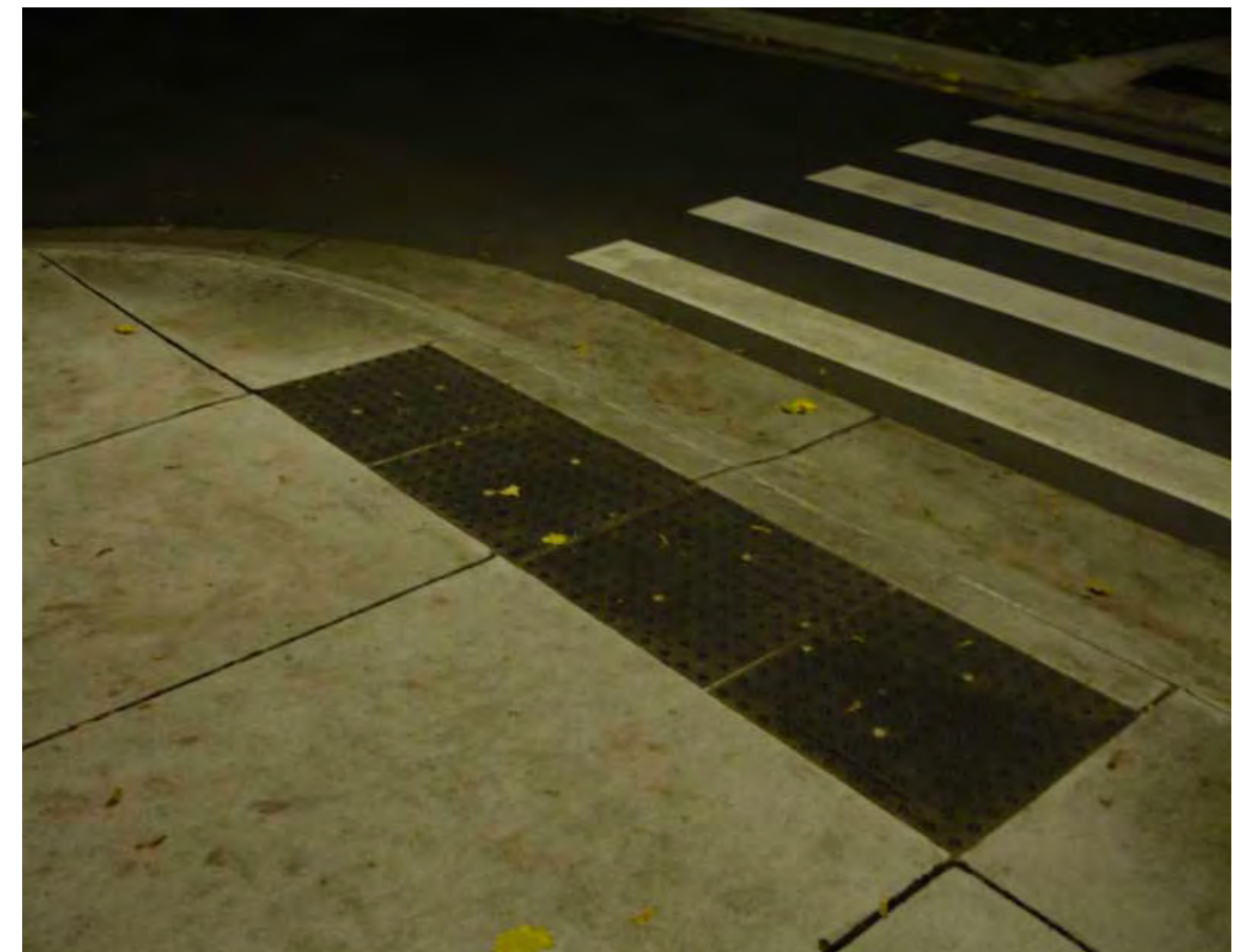
Curb ramp and crosswalk
